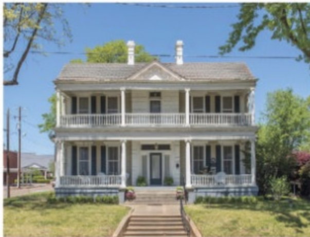
Richard Trimble & Associates, Inc. | Richard Trimble, ASID Category: Historical Renovation/Preservation, 1st place Category Group: Mixed Categories – Commercial or Residential
